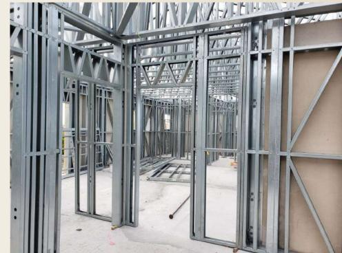
A lightweight galvanized steel structure is used for external walls and internal partition walls (frames) according to structural calculations for the building type. These models incorporate a steel (HRS) structure which is hot dipped galvanized to eliminate corrosion in salty environments.
